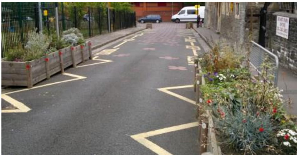
Figure 4: Illustrates the use of plant beds narrowing the local road to both detract vehicles and slow vehicle speeds (trafficchoices.co.uk, 2014).
